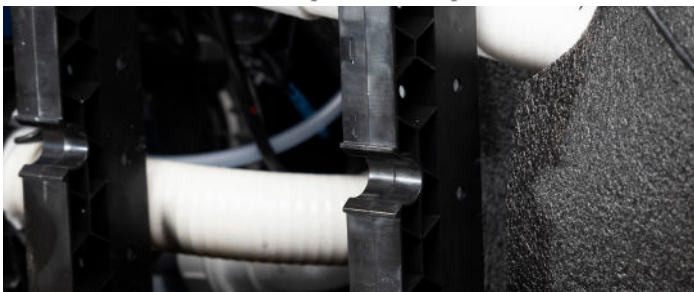
French Cleat (top) and C-Clip (bottom)
