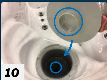
10 Insert the basket grill into the top of the filter, lining up the circular hole.
