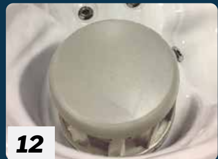
12 Replace the top lid by gently putting downwards pressure while turning clockwise, until it snaps back into place.
