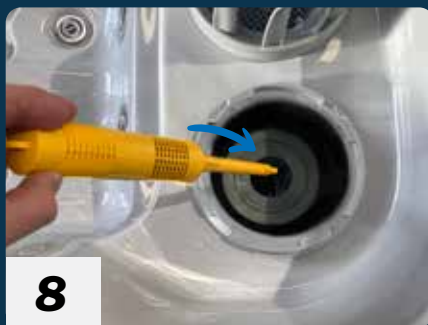
8 Place the Nature 2 Stick into the centre of the filter cartridge, extension tube first.
