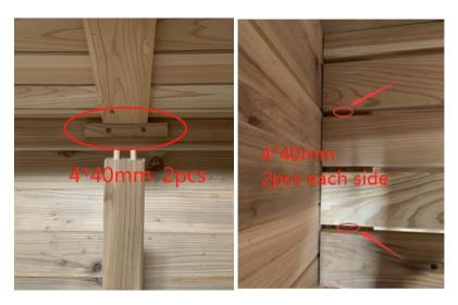
Install the bench leg supports on each side and secure with 2x '4\*40mm Screws'.
